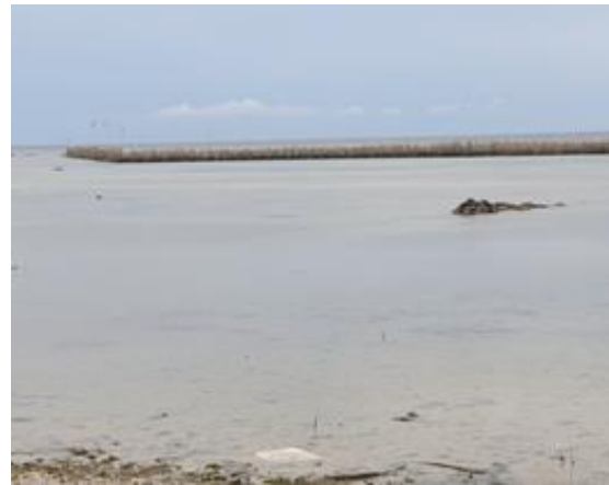
Figure 4. Sediment traps and wave attenuation in Bagongon
