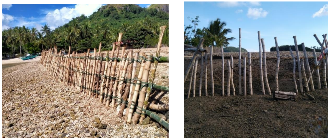
Figure 21. Bamboo posts used as slope protection to prevent erosion from the area of excavated berm
