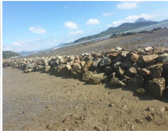
Figure 35. Constructed breakwater in Loong (Site 2)
