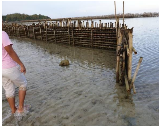
Figure 4. Sediment traps and wave attenuation in Bagongon
