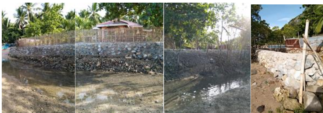
Figure 20. Completed slope protection in Tambaliza
