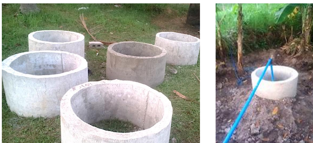
Figure 29. Installed deep well made from culverts for the NFS irrigation system
