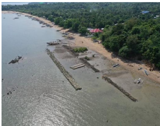
Figure 34. Drone view of the living breakwater installed in Loong (Site 1)
