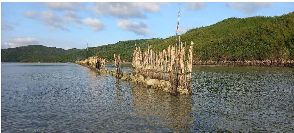
Figure 9. Stone reinforcement in the wave attenuation fence in Site 3 in Bagongon
