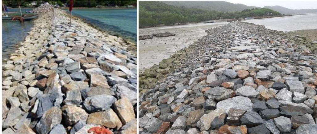
Figure 12. Low crest semi-permeable breakwaters in Purok Proper (left) and Purok Palina (right) in Bagongon.
