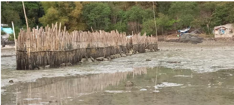
Figure 8. Stone reinforcement in the wave attenuation fence in Site 1 in Bagongon
