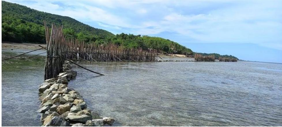
Figure 10. Stone reinforcement in the wave attenuation fence in Site 6 in Bagongon
