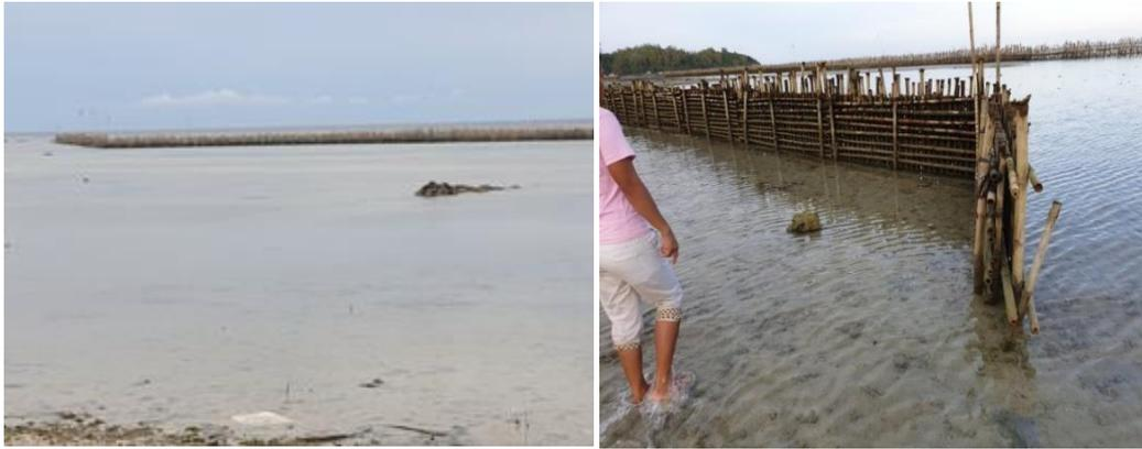
Figure 7. Wave attenuation fence (left) and sediment trapping fence (right).
