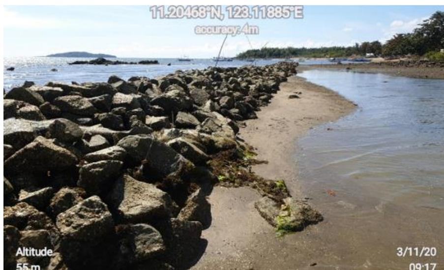
Figure 9. Sediment buildup around the breakwater in Site 1 in Loong in March 2020.
