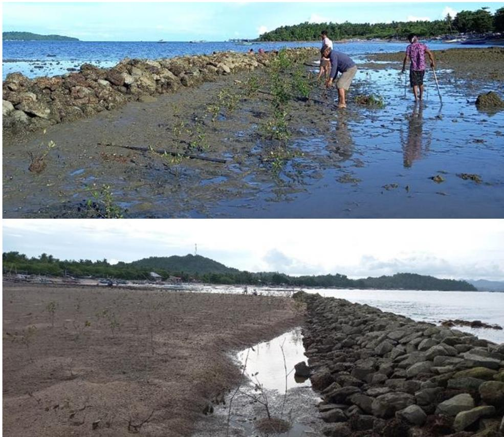
Figure 14. Mangrove seedlings planted on the accumulated sediment on the shore side of the breakwater in Sitio Mabinuligon (Site 2) in Loong.
