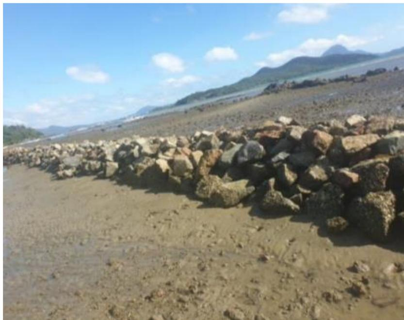
Figure 5. Semi-permeable living breakwater in Purok Mabinuligon in Loong (Site 2) that facilitated sediment accumulation favorable to mangrove planting.
