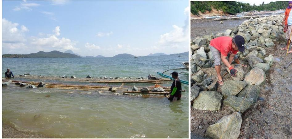
Figure 6. Transporting stones to breakwater construction site at high tide (left) and manual piling of stones at low tide (right).
