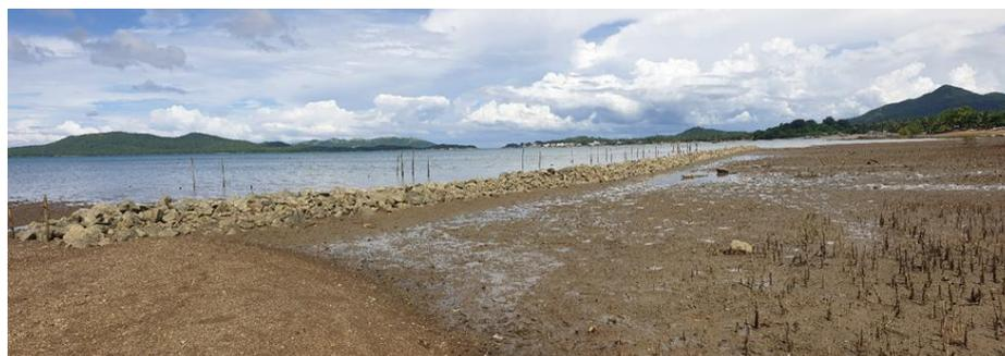
Figure 10. Sediment buildup on the shore side the breakwater in Site 1
