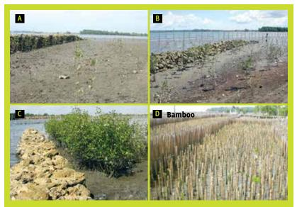
FIG. 14. Barriers made of a, b, c) rocks in Ermita, Dumangas, Iloilo (2007-2008), and d) bamboo support mangrove growth by reducing wave energy and trapping sediment.
