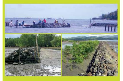
FIG. 15. Two lengths of breakwater, 0.9 m high by 1-2 m wide by 70 m and 110 m long, have consolidated sediment and provided both substrate and protection to planted and natural mangrove recruits in Pedada, Ajuy, Iloilo.
