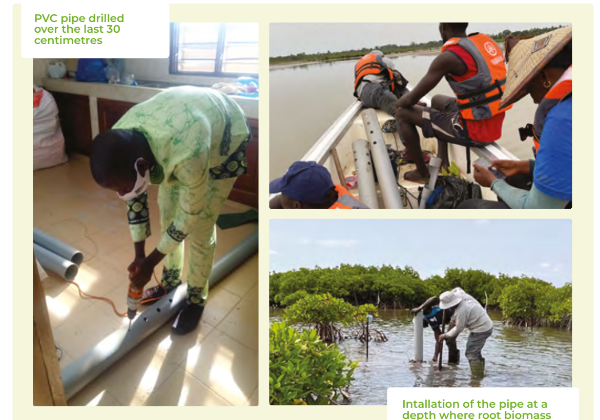
Figure 16. Installation of PVC pipes in reforestation sub-plots for collecting water samples and measuring physico-chemical parameters in situ , in accordance with Agraz Hernández et al. (2007). © C. Agraz Hernández
