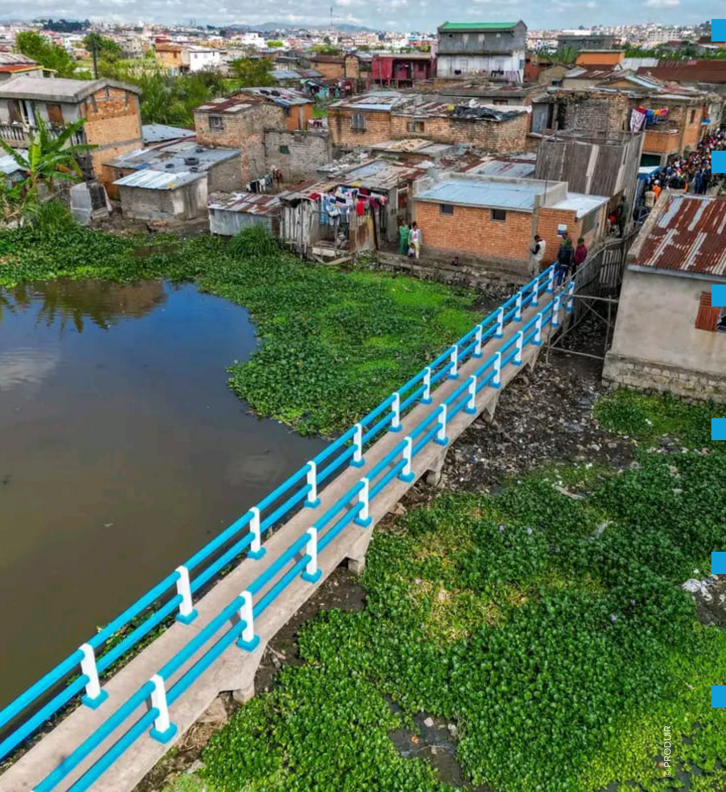
Image 35 : Construction of a footbridge as part of the PRODUIR project.
